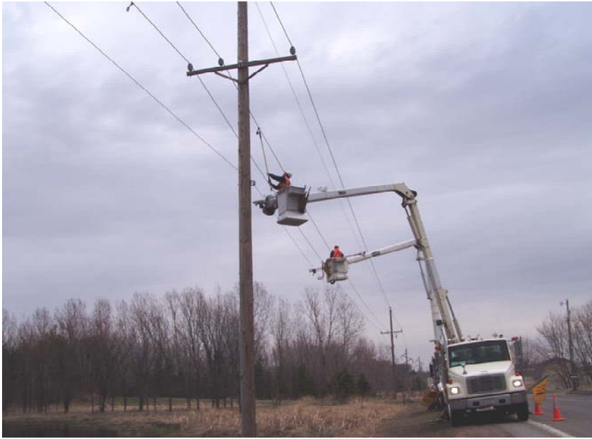
Figure 3. Local energy cooperatives and Xcel Energy install bird flappers on power lines.
